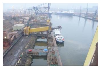
No. 2 Quay at Teesdock is the main hub for potash exports around the world, as well as various other bulk cargos. The structure enables seafaring vessels with storage capacities of some 33,000 tonnes to dock in order to load/unload cargo & bulk materials. For this reason the Quays ability to function is vital to the clients operations.
